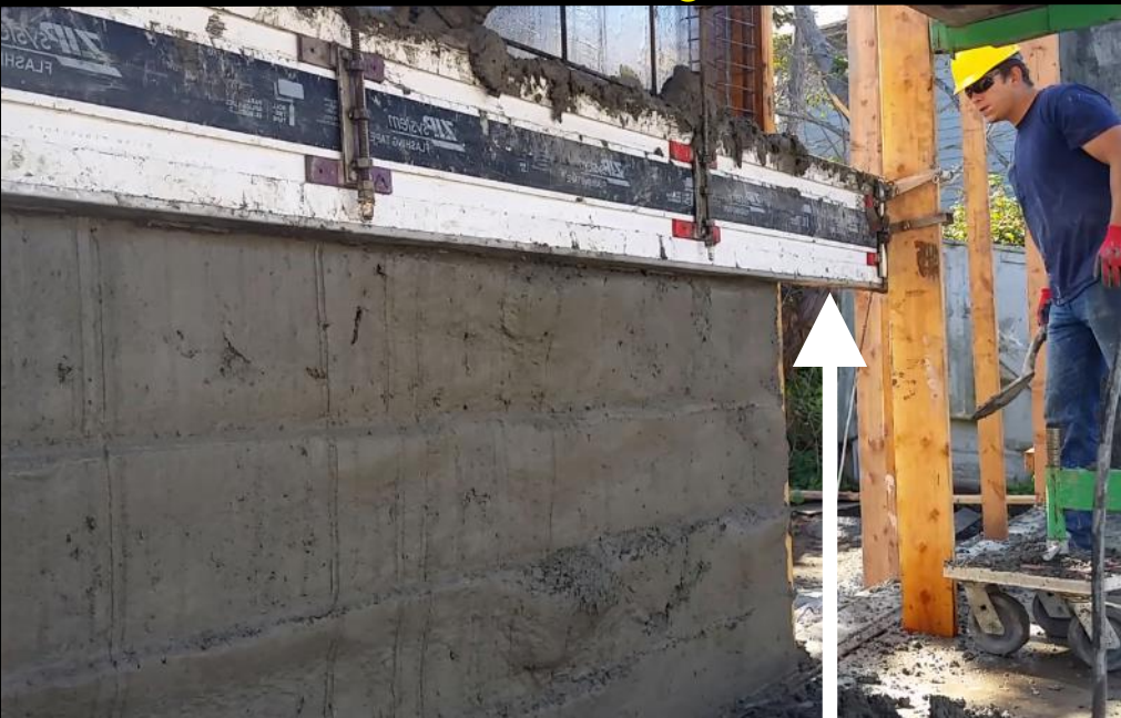
slip-cast vertically as fast as a foot per minute
