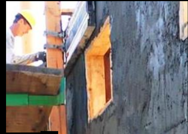
13' lift of fresh concrete →
