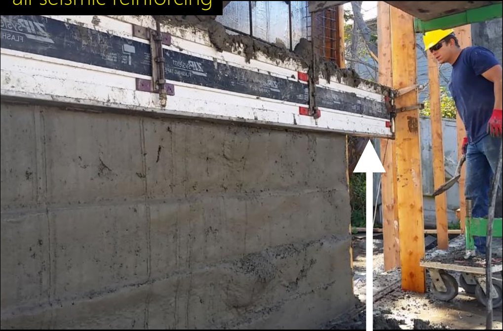
slip-cast vertically as fast as a foot per minute
